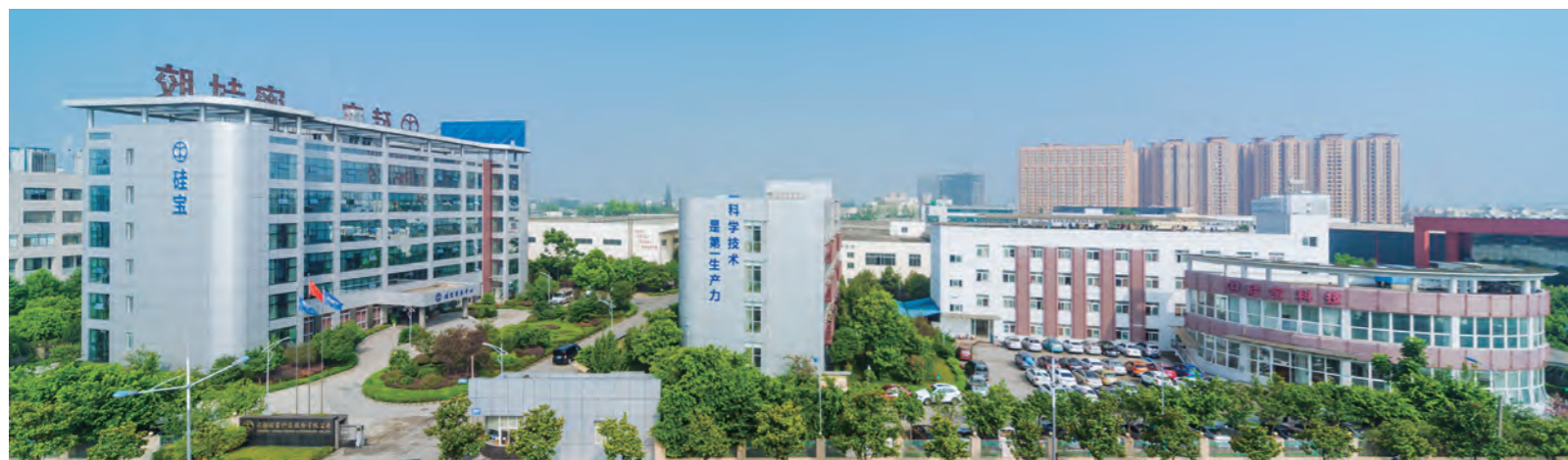
GUIBAO headquarter production base - Chengdu High-tech zone
