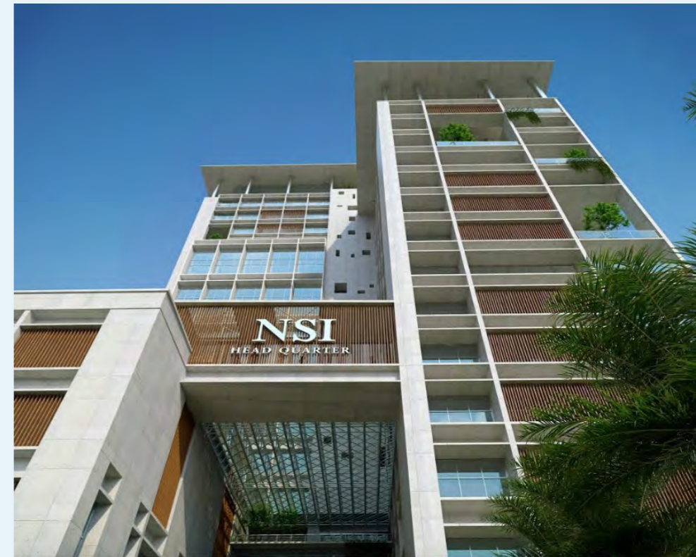
Project: NSI HEAD QUARTER Area: 6,500 m 2 Location: Dhaka, Bangladesh Product : GUIBAO 557 NEUTRAL SILICONE SEALANT FOR WINDOW AND DOOR GUIBAO 998 SILICONE WEATHERPROOFING SEALANT
