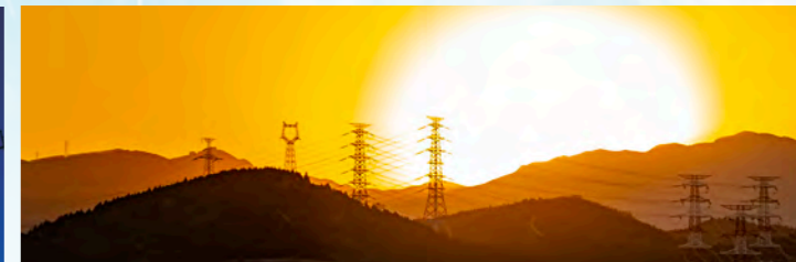
Uhv Transmission and Transformation
